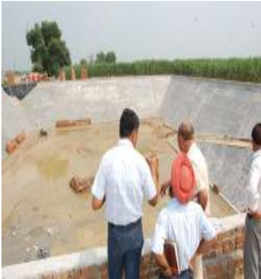
Community Pond (Under Construction) at Abohar
