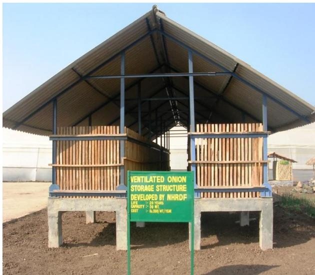
Improved storage structure developed by NHRDF
