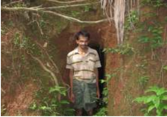
View of ' Surangam' an indigenous method of tapping spring water through tunnels
