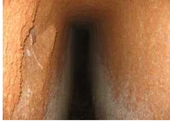
View of ' Surangam' an indigenous method of tapping spring water through tunnels
