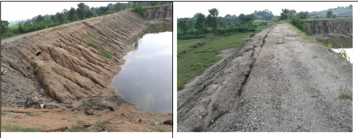
The tank did not have any lining as a result of which heavy soil erosion of embankment was taking place. The NGO was contacted over phone and asked to repair the tank and provide lining material, as stipulated in NHM guidelines, which was agreed to.
